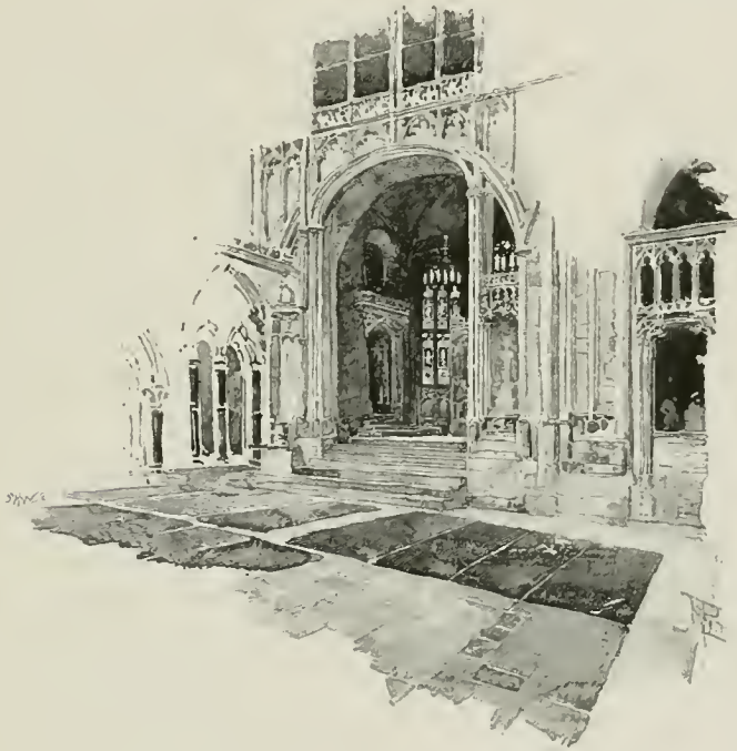
ST. PAUL'S CHAPEL, NORTH ARM OF TRANSEPT.
